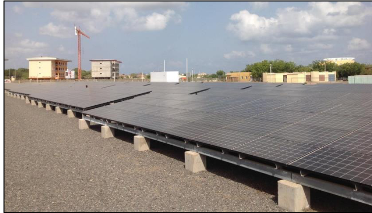
Fig.1. PV system installation
